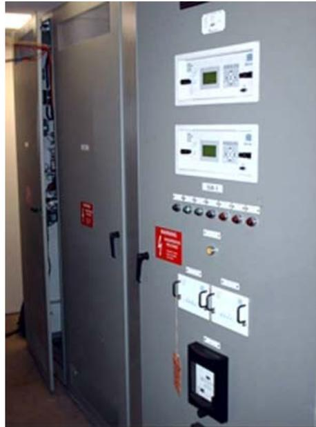
Figure 9. Cabinet with Redundant Digital Excitation Control Systems
