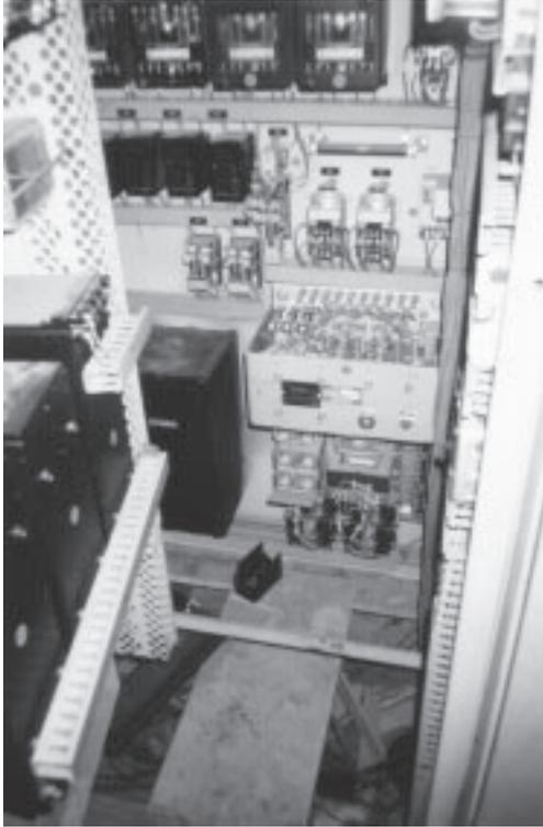
*Figure 6: Automatic Voltage Regulator Gas Turbine-Generator unit.*
