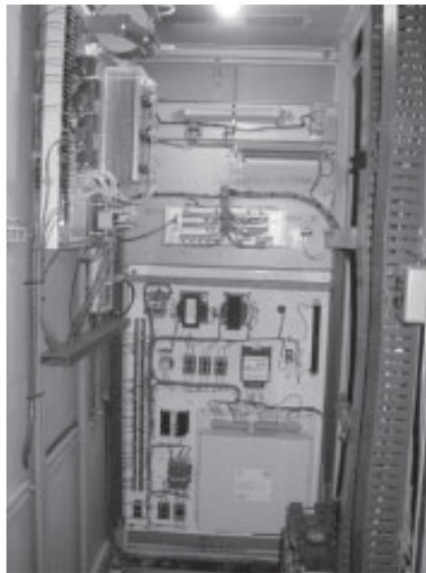
Figure 13: Retrofit of a new digital voltage regulator system into SCT-PPT excitation switchgear lineup.
