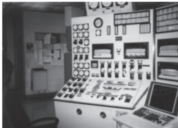
*Figure 11: Existing generator controls and metering located at the BTG control panel are interfaced to the new digital control system.*
