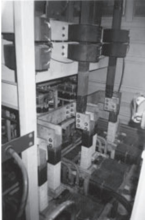
*Figure 2: SCTs and linear reactors located on the Generator Neutral Bus.*
