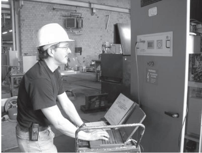
*Figure 14: Start-up and commissioning of the new digital voltage regulator system is easier with all adjustments for setting the generator response, limits, protection, etc. at your fingertips via the serial port connection to your laptop computer.*
