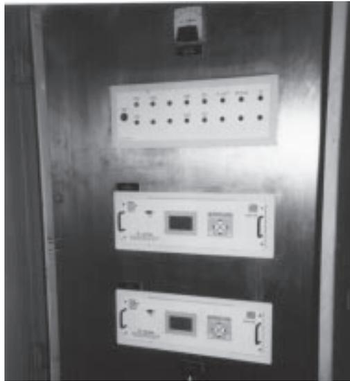
*Figure 10: Dual digital control modules with automatic transfer and a local alarm/status LED*
