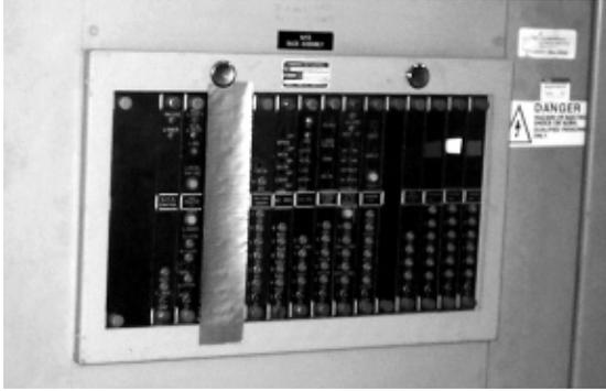
Fig. 1. Bus Fed Analog Voltage Regulator
