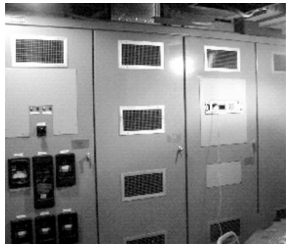
Fig. 14. The lineup of the OEM's original equipment. The digital controller is installed on front of cabinet door.
