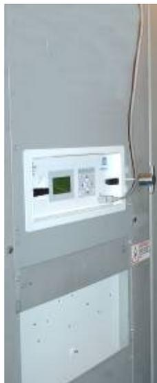
Fig. 4. Digital Controller installed in Cabinet Door
