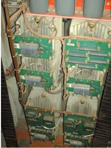
Fig. 2. Existing 3 SCR, 3 Diode Half-Wave Bridge
