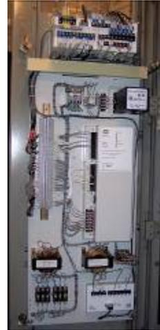
Fig. 5. Back door of Digital Controller panel showing Firing Circuit and related hardware
