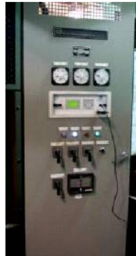
Fig. 13. New front door provided with new cutouts for digital controller. A serial cable is used for a laptop connection.
