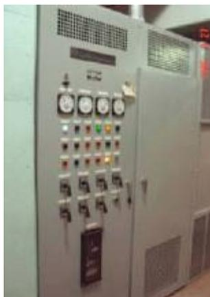
Fig. 12. Using the analog technology: Many lights, switches and meters on front of doors of OEM equipment
