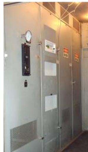
Fig. 6. Exciter cabinet lineup with Digital Controller installed
