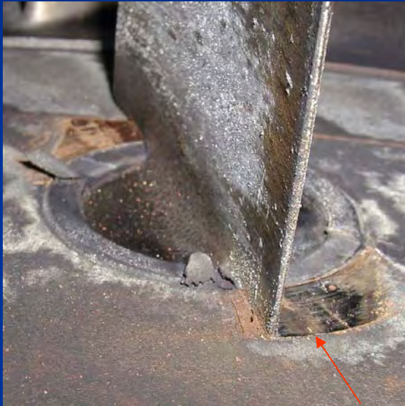
Variable Inlet Guide Vane Rubbing Against Inlet Bellmouth
