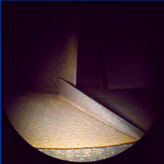
Stage S-1 Shim Protruding Into Air Path
